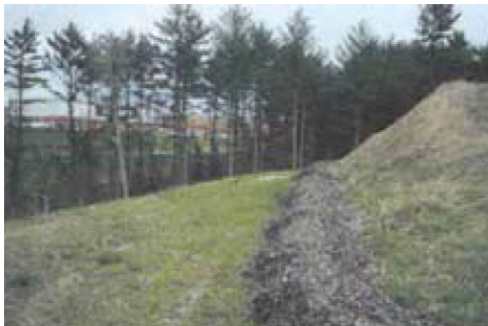
Figure 5. Ground wood waste being used in a berm for erosion and sediment control.
