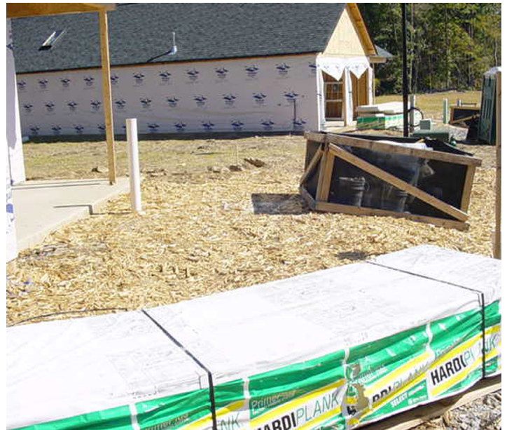
Figure 4. Ground wood waste used for a delivery pad.
