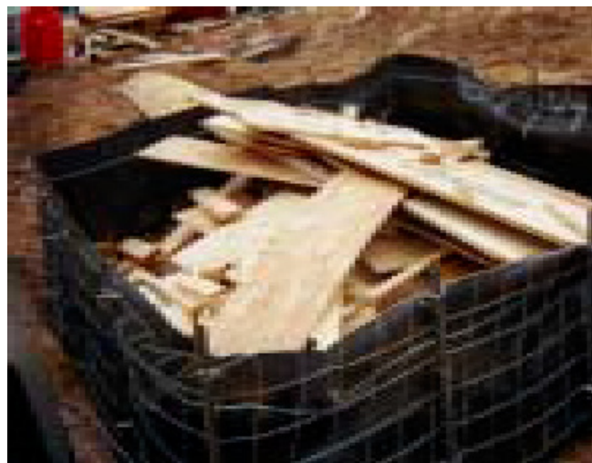
Figure 3. Example of a wood waste storage area.
